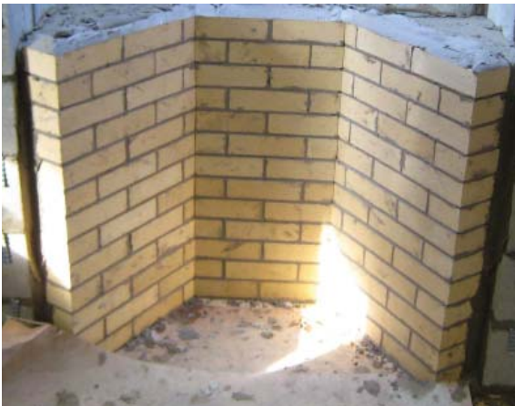
Figure 6. Completed Firebox Wall Construction
