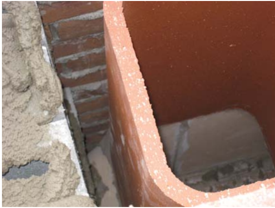
Figure 15. Starting the Chimney from Smoke Dome
