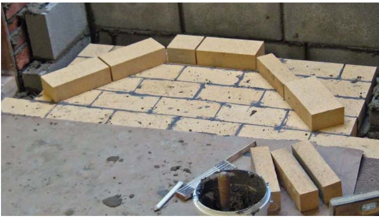
Figure 4. Interior Hearth Rough Layout
