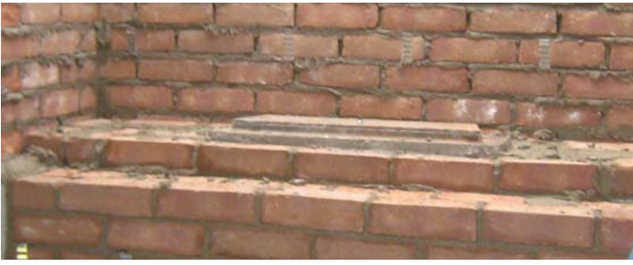
Figure 11. Setting the Damper
