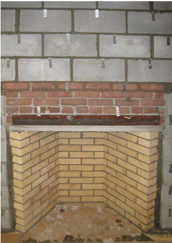
Figure 17. Fireplace Ready for Surround Installation
