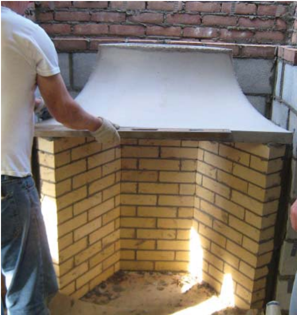
Figure 8. Setting the Rumford Throat
