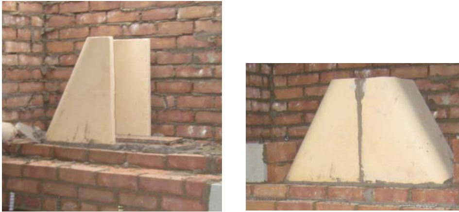
Figure 13a and 13b. Setting the Smoke Dome
